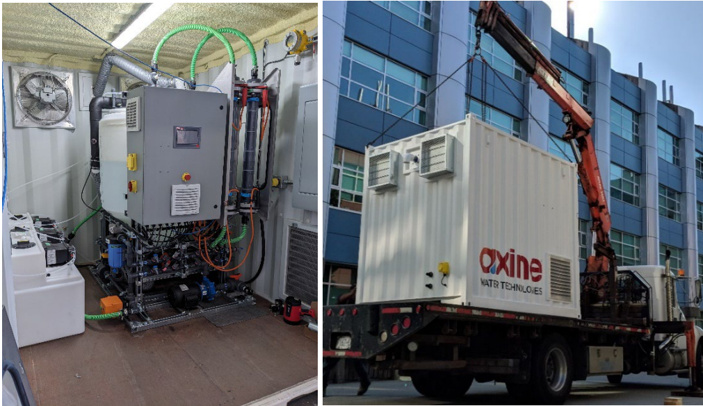
Figure 4. Axine's Pilot-scale Test System
