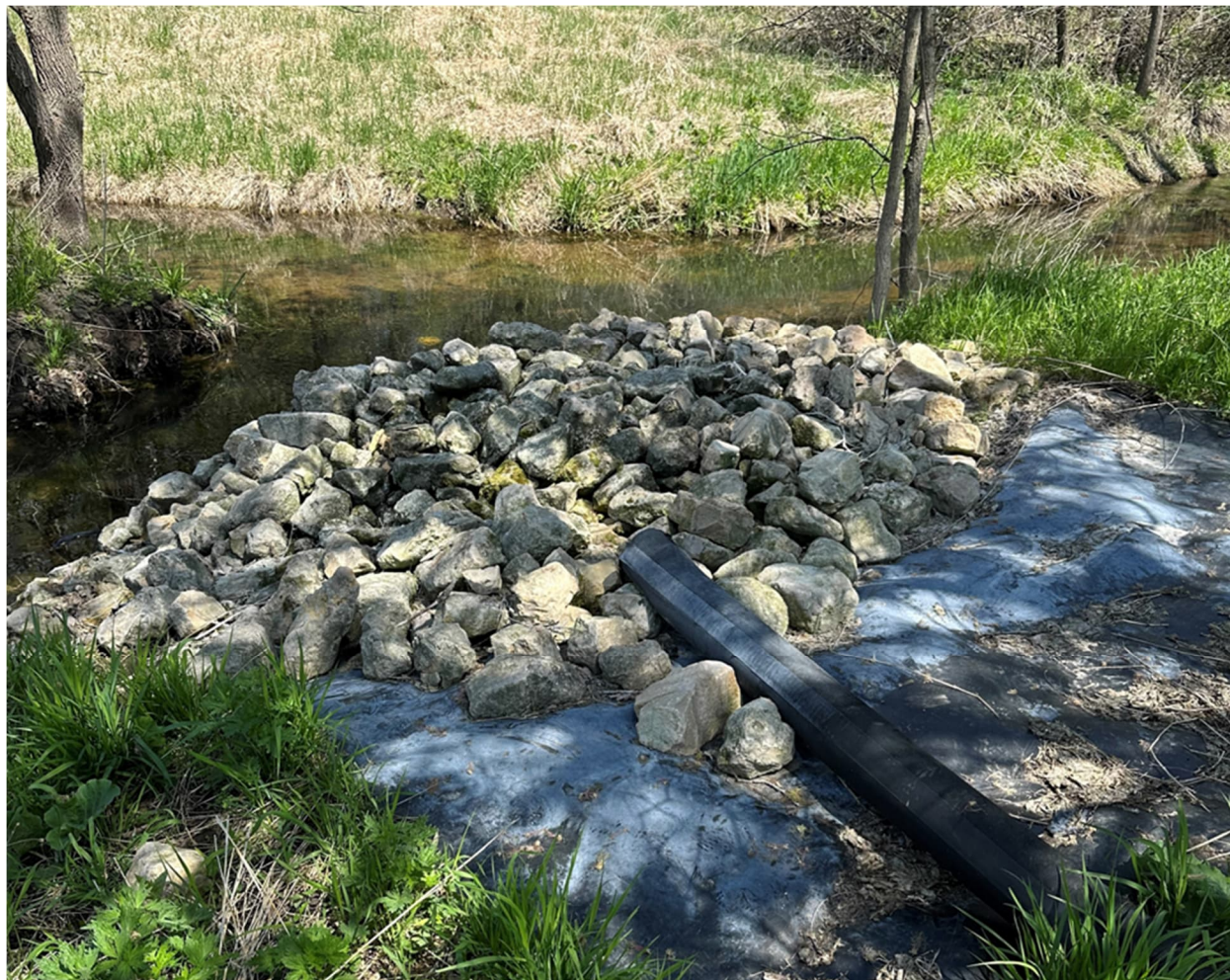
Figure E.4: Treated Effluent Discharge Location and Erosion Control Structure.
