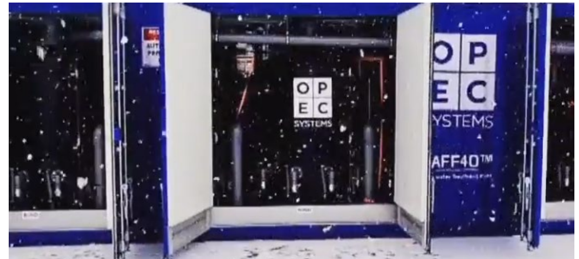
40-ft OPEC system for landfill leachate treatment in Sweden
